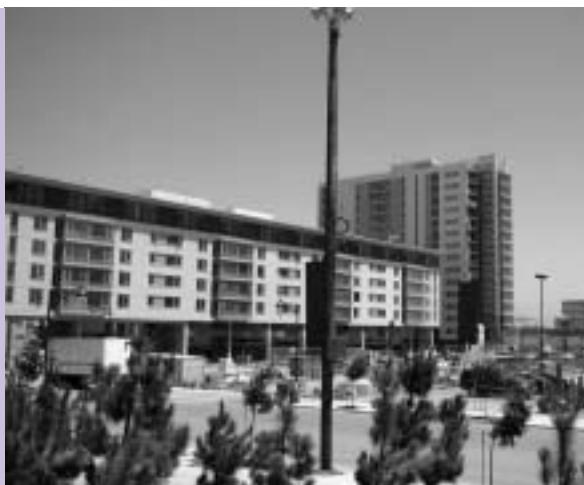
UCSF's campus housing complex defines an internal courtyard. Shown here is the South building.
