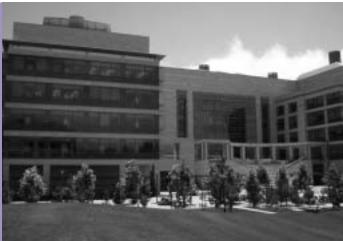
QB3 (left), Genentech Hall, and their monumental entry porch.
